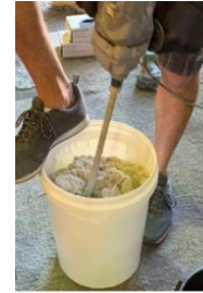
Mixing Epoxy Mortar
