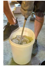
Mixing Epoxy Mortar
